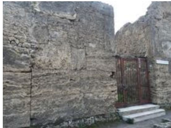
Fig. 9 Travertine opus quadratum façade, House of Orpheus, Pompeii
