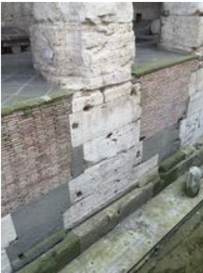
Fig. 8 Travertine foundation stones under the remains of the Temple of Hadrian, Rome
