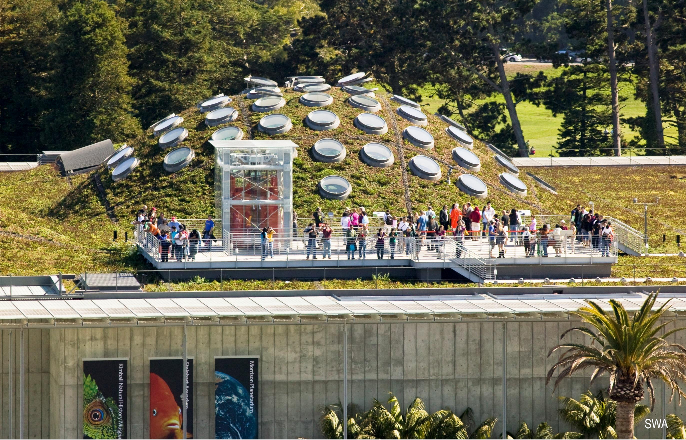
Green roof at California Academy of Sciences
