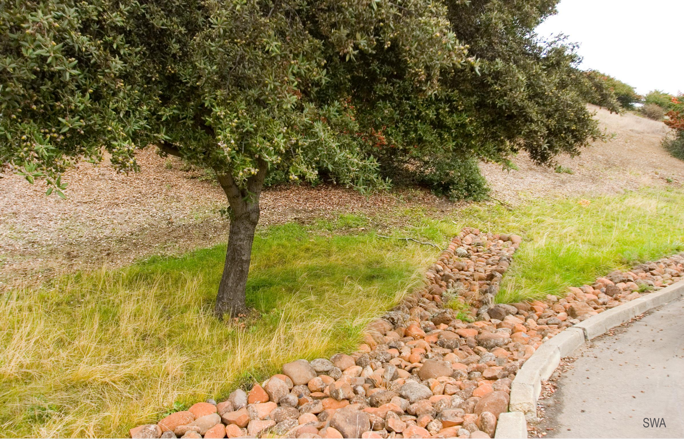
Stormwater and erosion control at CSU East Bay
