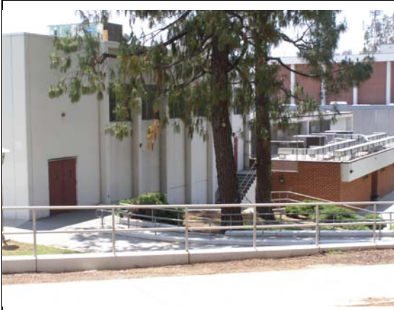
Image 3. View of upper/north level of west facade looking southeast.
