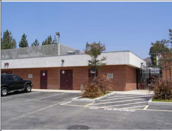
Image 1. View of south and east façades of Building 27B looking southwest.
