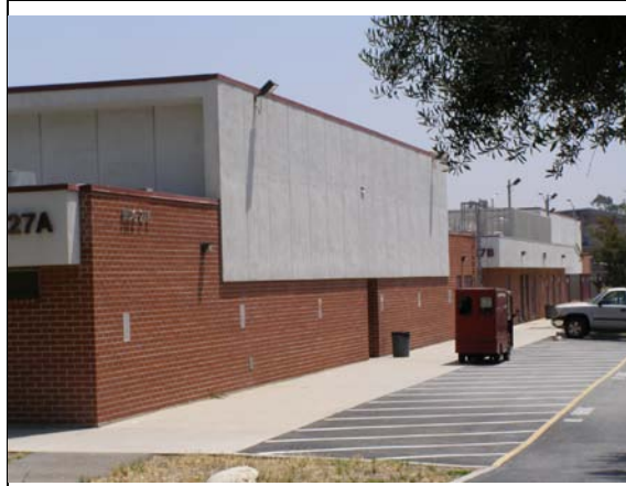
Image 4. View of south facade looking northeast.
