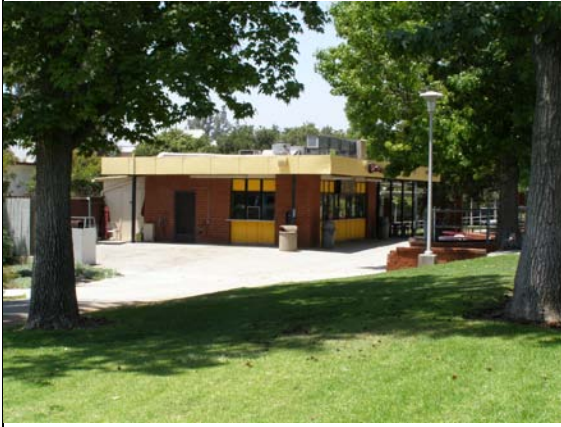
Image 1. View of north and west facades looking southeast.
