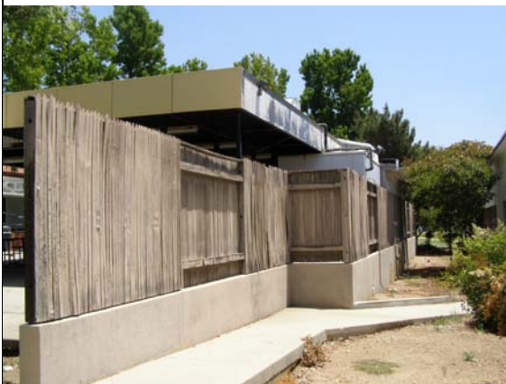
Image 5. View of south facade looking northeast.
