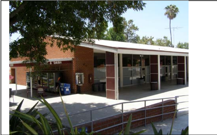
Image 1. View of north and east facades looking southwest.
