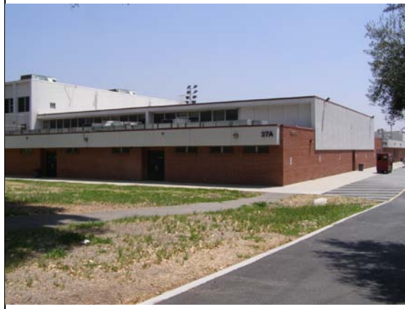
Image 2. View of lower/southern half of west and south facades looking northeast.
