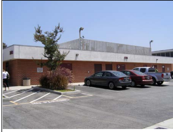
Image 2. View of south façade of Building 27B looking northeast.
