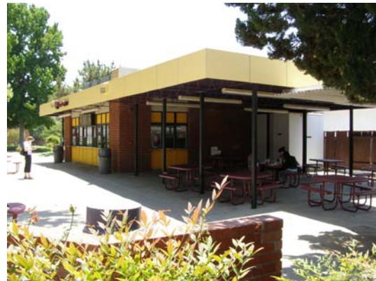
Image 4. View of north and east facades looking southwest.
