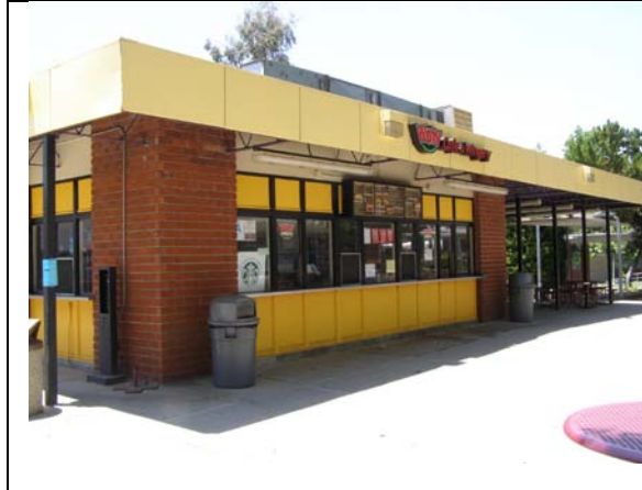
Image 2. View of north facade looking southeast.
