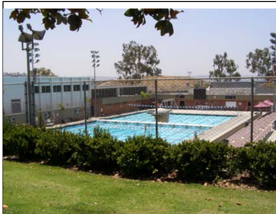
Image 4. View of pool and north façade of Building 27B looking south.
