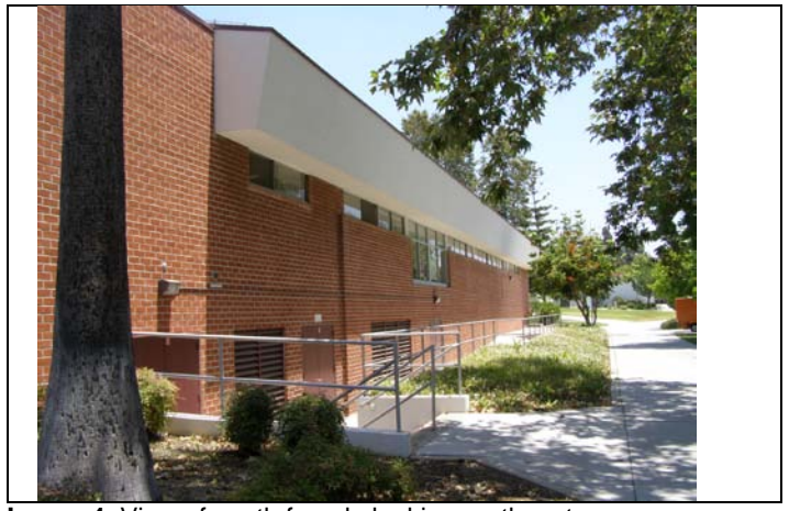
Image 4. View of south facade looking northeast.
