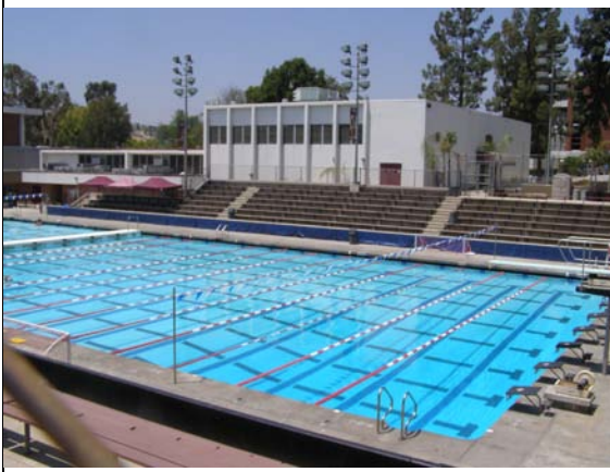
Image 1. View of north and east facades looking southwest.
