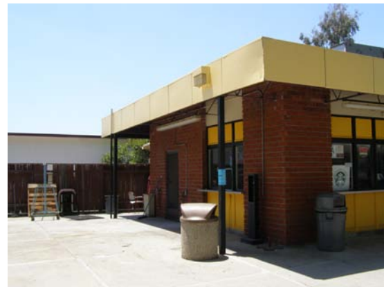
Image 3. View of west facade looking southeast.
