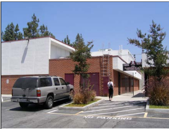
Image 5. View of south and east facades looking northwest.
