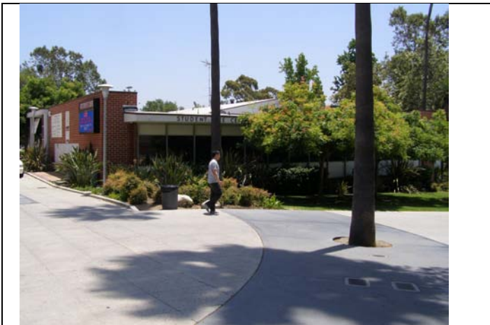
Image 3. View of north and west facades looking southeast.
