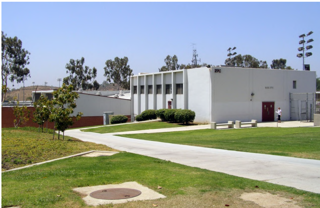
Figure 6. Locker Rooms (27C)
